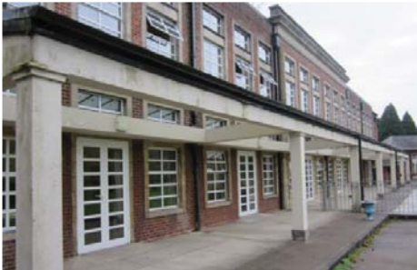
(fig.162) SAINT DAVNET'S HOSPITAL Armagh Road Monaghan (1937-42)
