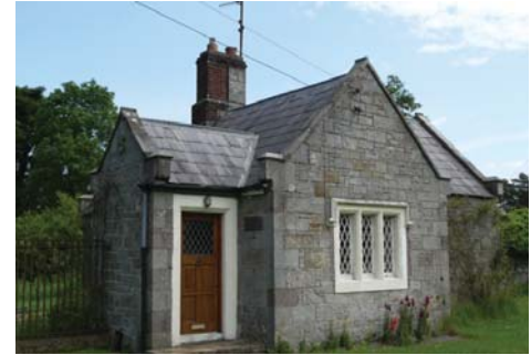
(fig.73) LAKE LODGE Lough Fea House Losset (c. 1845)
