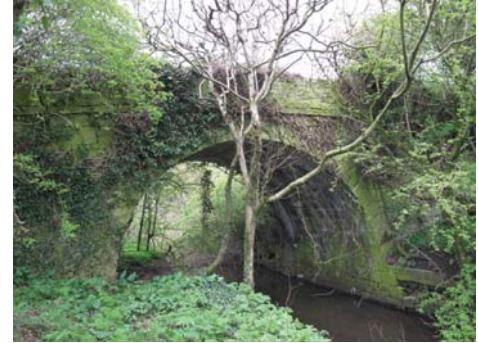
(fig.42) PIPER'S BRIDGE Killeef (c. 1840)
