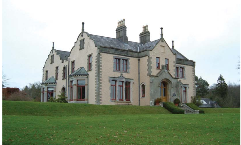
( fig.114 ) ANNAGHMAKERRIG HOUSE Mullaghmore (c. 1860)
