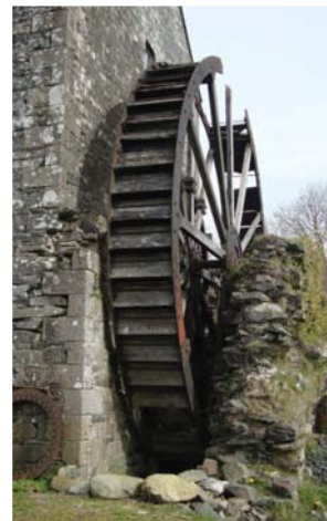
( fig.45 ) TULLYGILLEN MILL Tullyard (c. 1850)
