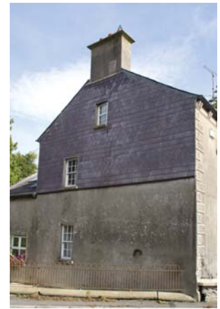
W. SLOAN Decorative slatehanging adds to the architectural interest of Sloan's house at Swann's Cross.
