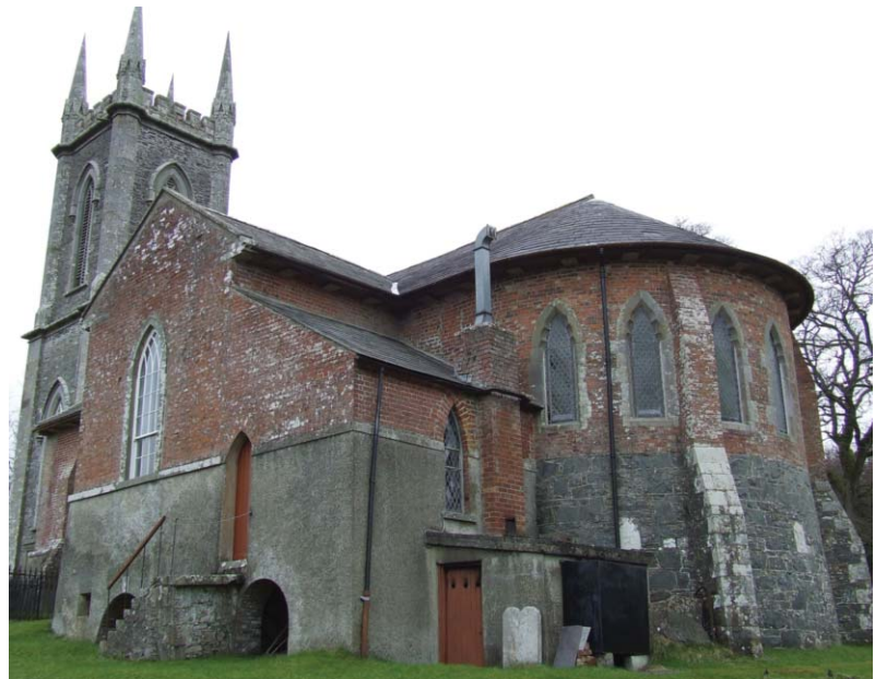
( fig.13 ) SAINT JOHN'S CHURCH Dawson Grove Demesne (1729, altered 1771, 1815, 1840 and 1870)
