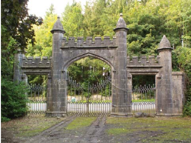
(fig. 68) THE GOTHIC LODGE Mullyjordan Glaslough (c. 1812)
