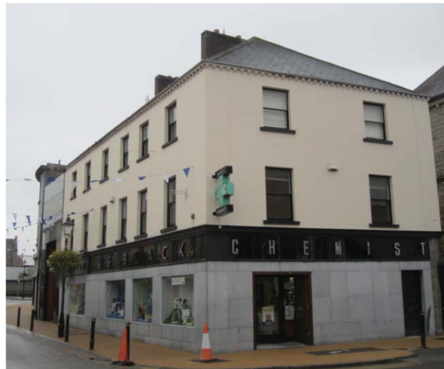
(fig.163) W.S. BLACK Mill Street Monaghan (c. 1830, with later shopfront)
