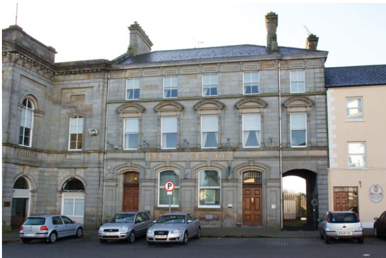
( fig. 92 ) BANK OF IRELAND The Diamond Clones (1892)
