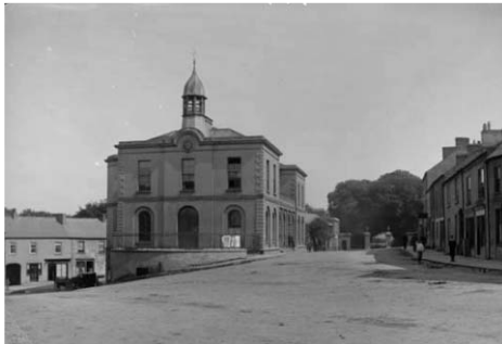
CASTLEBLAYNEY MARKET HOUSE/COURT HOUSE Market Square Castleblayney (c. 1790, 1856)
