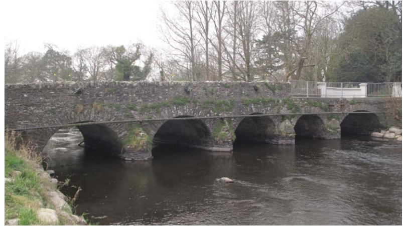
( fig. 38 ) INISHKEEN BRIDGE Inishkeen Glebe (1801)
