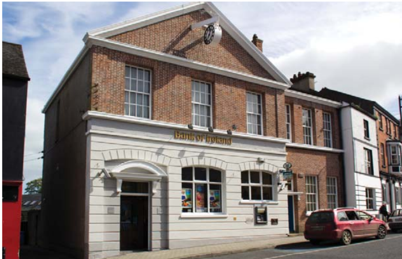
(fig.147) BANK OF IRELAND Main Street Upper Ballybay (1926)
